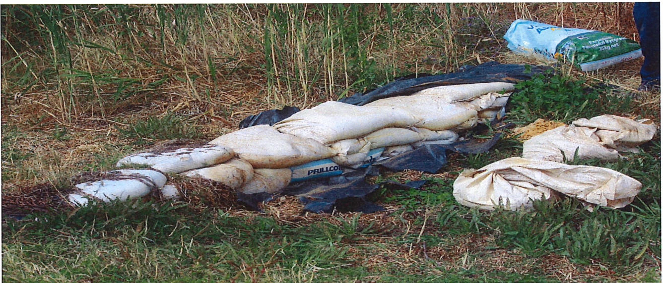
Drain blocks constructed to hold back water in old drainage systems
